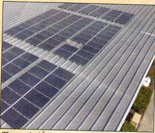
The roof of Solar Direct HQ
