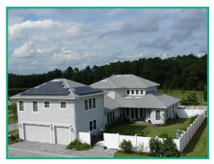
• 4.8 KW Grid-connected PV
